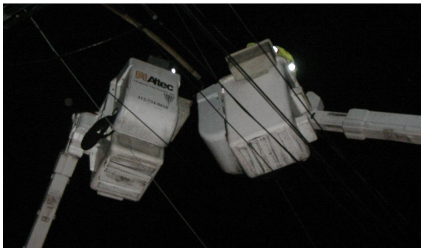
Figure 6. Trucks Used to Replace Streetlights [12]
